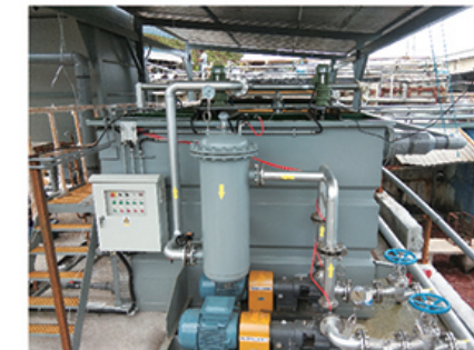
2. Model: GDXF-60T Capacity: 60m 3 /h Wastewater type: chicken slaughterhouse wastewater Location: Malaysia
